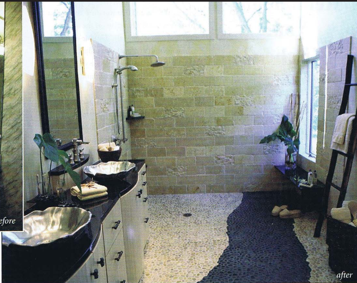
The Benike's new bathroom includes an open shower accented by limestone bricks and a heated stone pebble floor.
